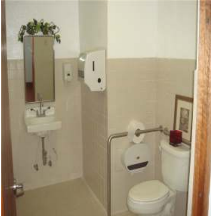
Remodeled ADA Compliant Restroom
